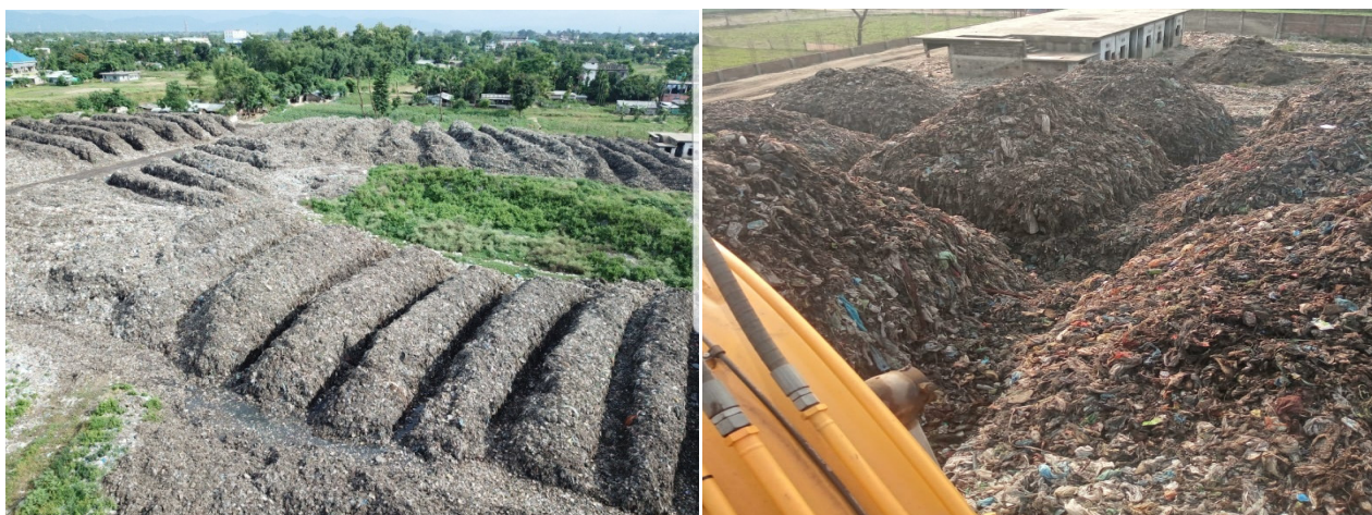
Picture 3: Aerial view of Dimapur Municipal Council waste dump site in-process Bioremediation
