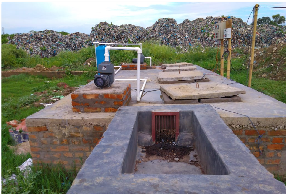
Picture 2: Construction of Septage Management Plant at Burma Camp, Dimapur
