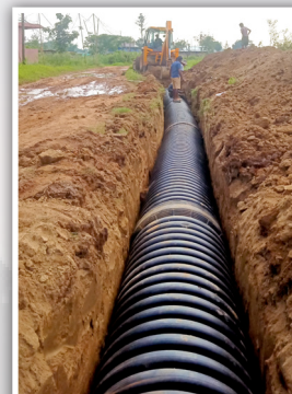
Laying of the main sewer trunk
