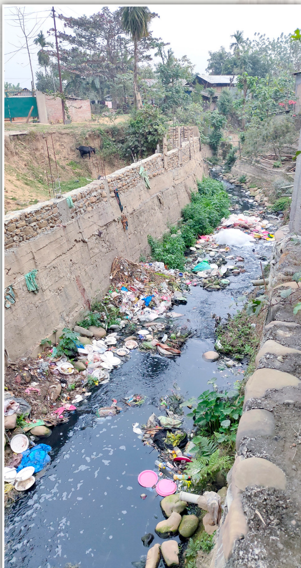
Hospital Nullah (upstream)
