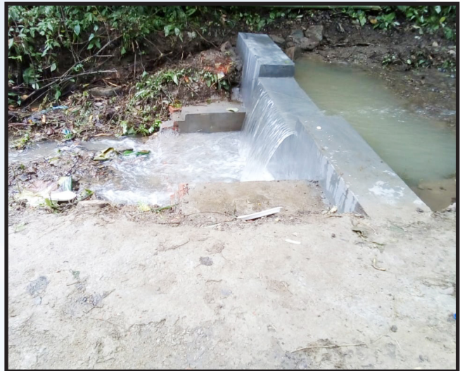
Waterhole cum Water Harvesting Structure at Yonchucho and Tsingiki village
