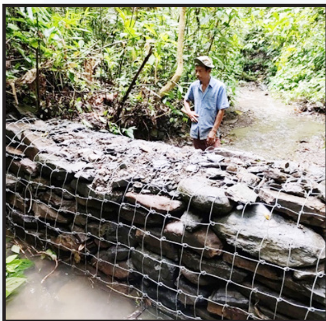
Gully plug at Yaksokyu stream
